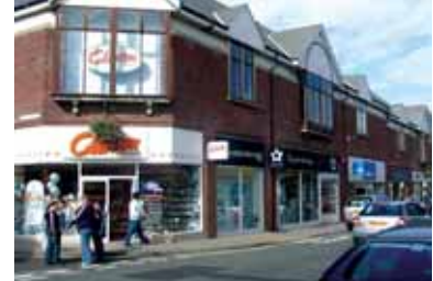
1-4 RITZ SHOPPING CENTRE, WORKINGTON, CUMBRIA
